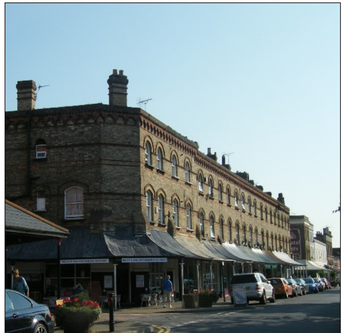
The first row of shops that were built in Station Road in the late 1870s. It is thought most likely that this row of shops was designed by Charles Nightingale Beazley. Compare this photograph, taken in September 2012, with second row of shops that were designed by William Henry Lockwood illustrated on page 4 of this Newsletter
