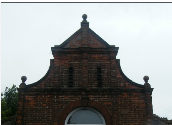
The matching 'Queen Anne Revival' gable at the western end of the former St Saviour's School, Elm Grove
