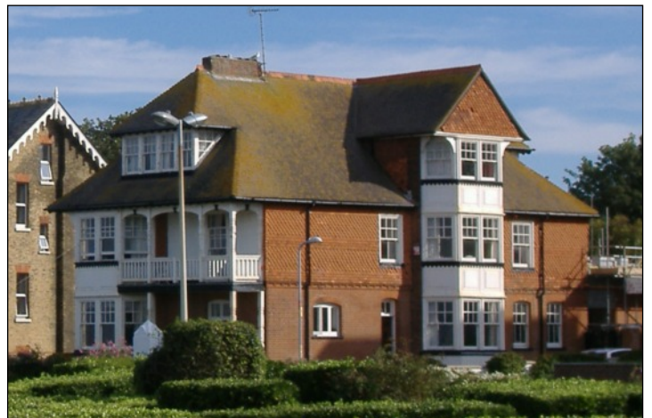
Penrhyn (formerly Penrhyn Lodge), Sea Road photographed in September 2005 shortly after the commencement of the large rear extension
