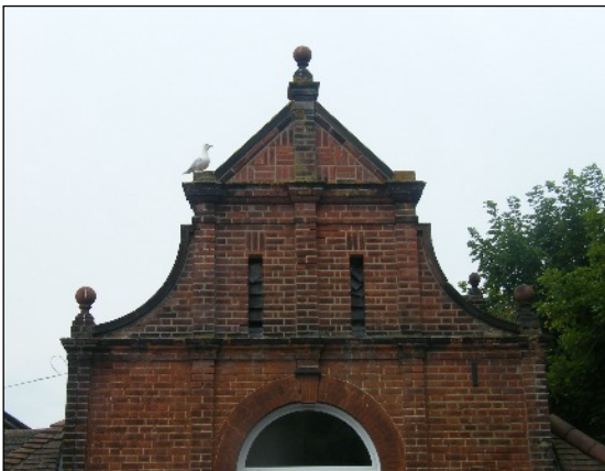
The 'Queen Anne Revival' gable at the eastern end of the former St Saviour's School, Elm Grove Note the decorative brickwork in front of the seagull
