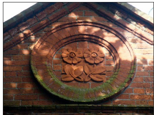
A pair of terracotta sunflowers within a circular moulded red brick circular surround at one of the house's many gable ends
