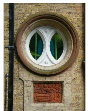
The attractive round window above the terracotta date panel to the left of the front entrance
