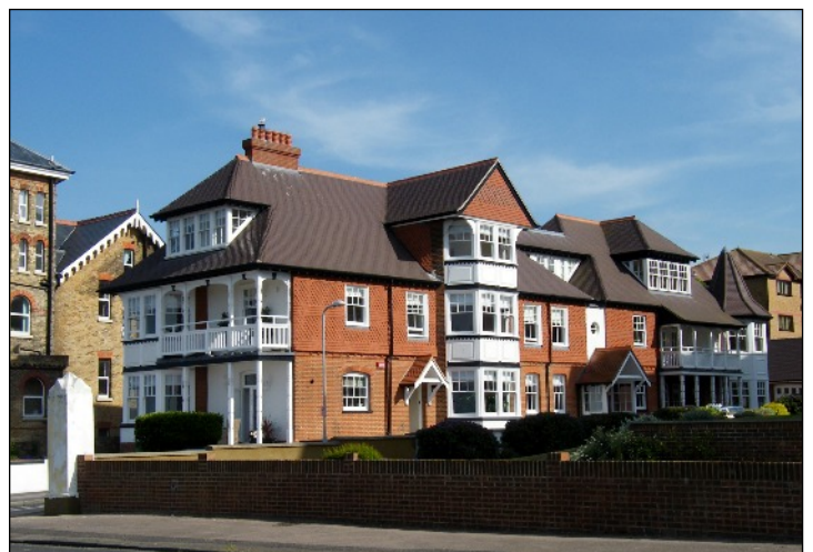
Penrhyn photographed in June 2011 after the completion of the rear extension
