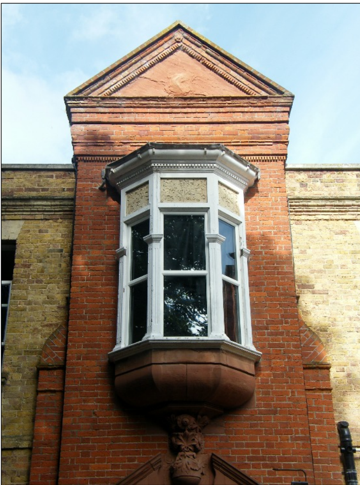
The oriel window above the front door with three sgraffito panels. It would appear from this photograph that there had, at one time, been some form of terracotta decoration - possibly the Hatfeild family crest - contained within the pediment
