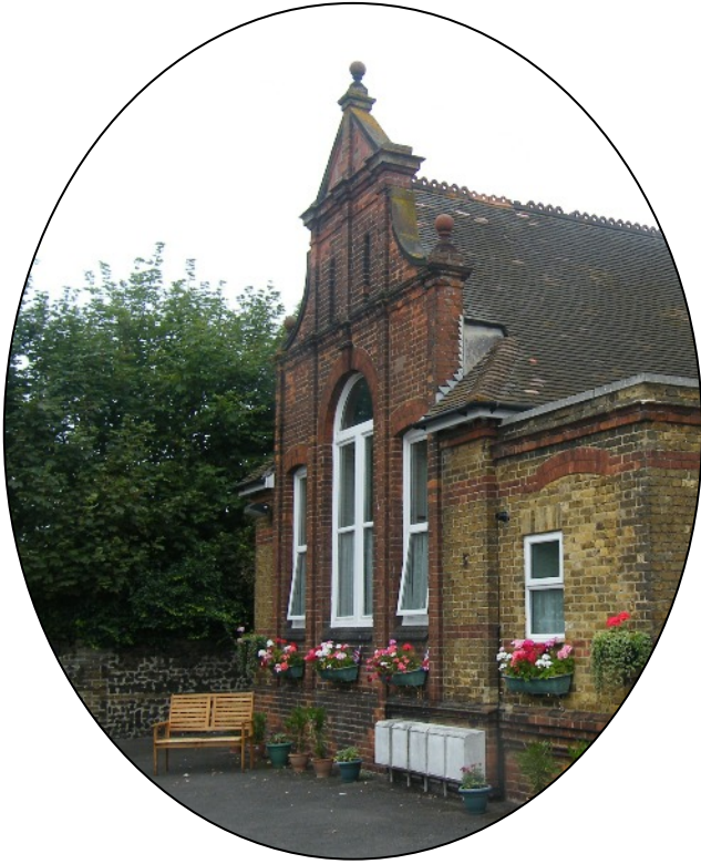
The eastern end of the former St Saviour's School (now apartments), Elm Grove, Westgate-on-Sea
